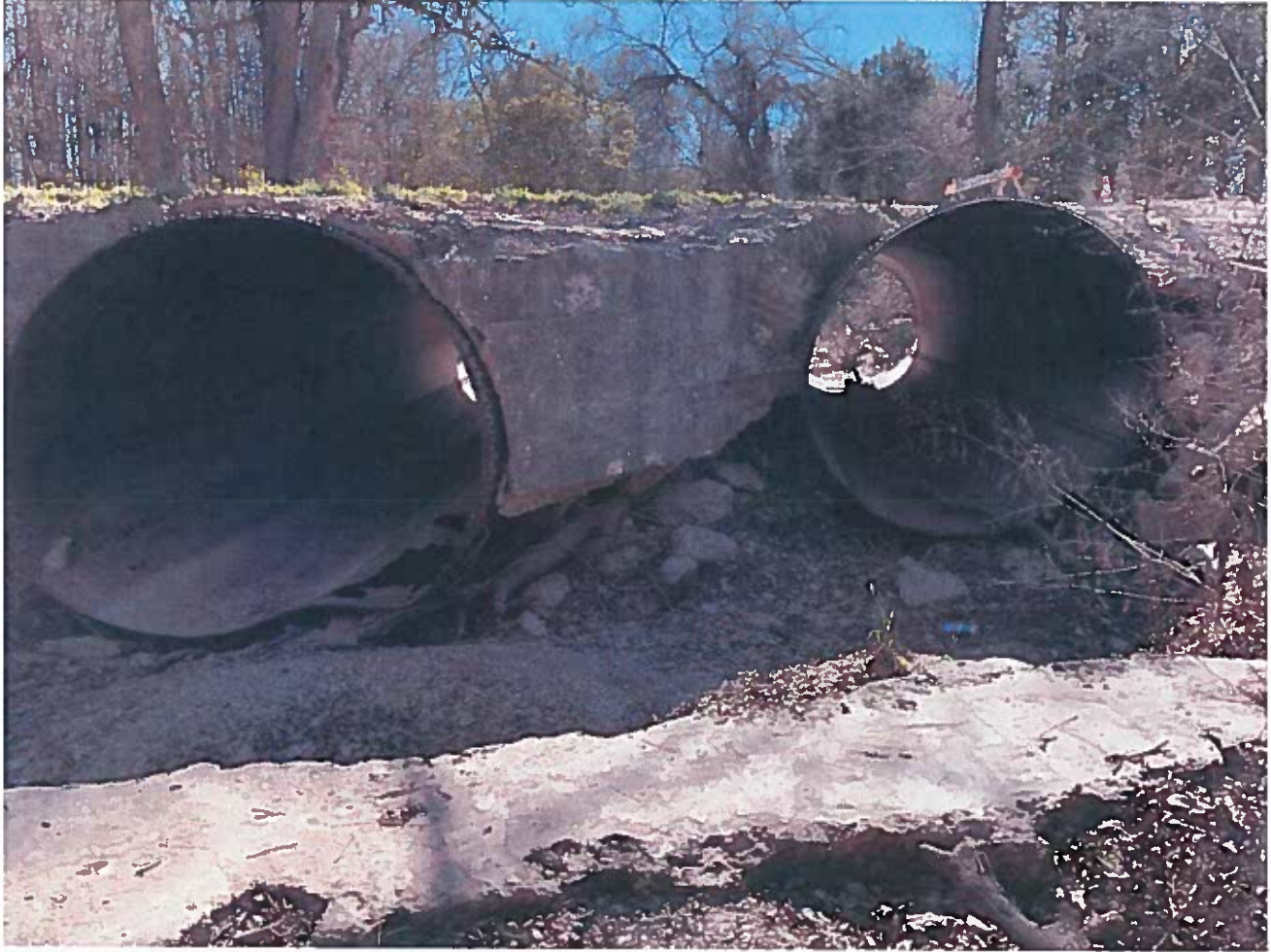
View from Downstream (note apparent hollow areas behind concrete and around pipes)
